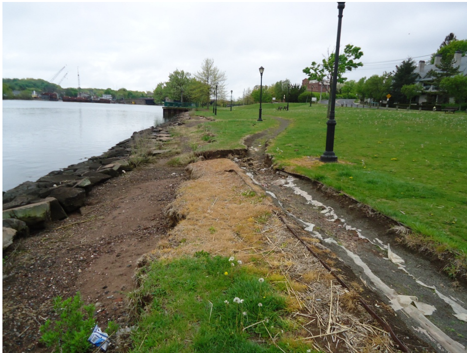
Figure 4-2. Shoreline Erosion and Erosion on Walkways at Quinnipiac River Park
