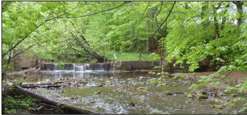
Figure 4-26. Small Dam on Wharton Brook
