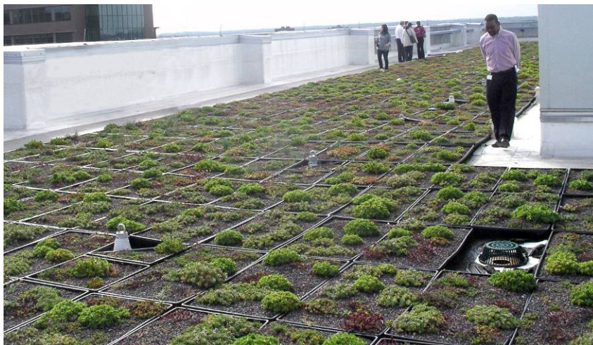
Figure 4-9. Modular Green Roof System Installation
